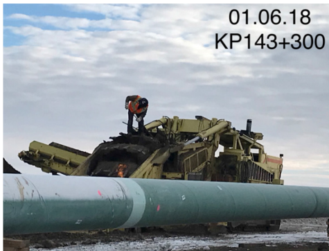
3. Ditcher maintenance – Km 143+300 – Jan 6, 2018
