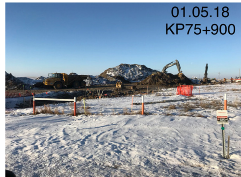
4. Tie-in – km 75+900 – Jan 5, 2018
