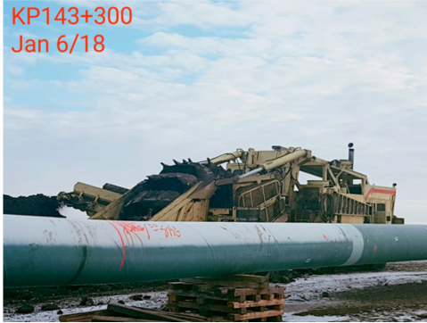
7. Ditcher – Km 143+300 – Jan 6, 2018
