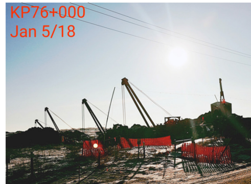
2. Tie-in – Km 76+000 – Jan 5, 2018
