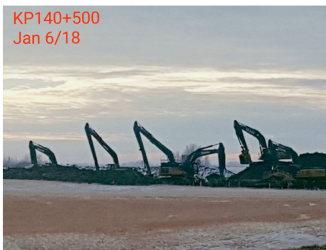
5. Backfill – Km 140+500 – Jan 6, 2018
