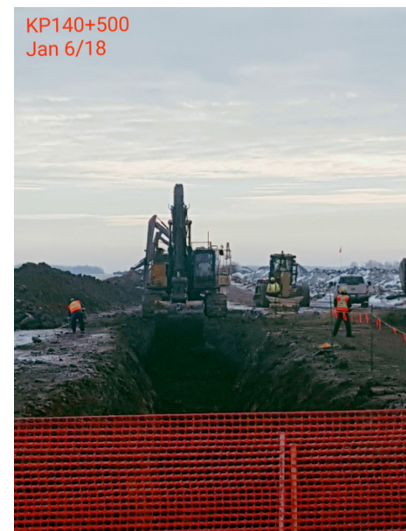
6. Mainline lowering in - Km 140+500 – Jan 6, 2018
